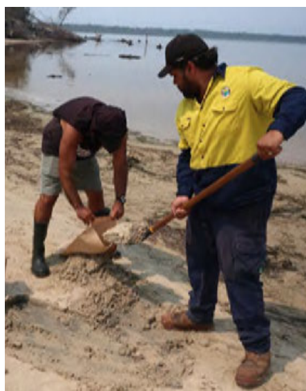
Rob Hudson GEGAC (left) and Max Solomon GLAWAC filling sandbags for the wall that will give the dunes instant short term protection until the sand is dredged.
