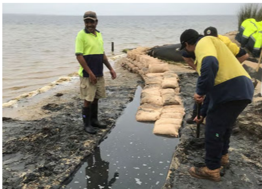
Ivan Hood from GEGAC (left) and Max Solomon from GLAWAC placing sandbags to form the sand bag barrier.
