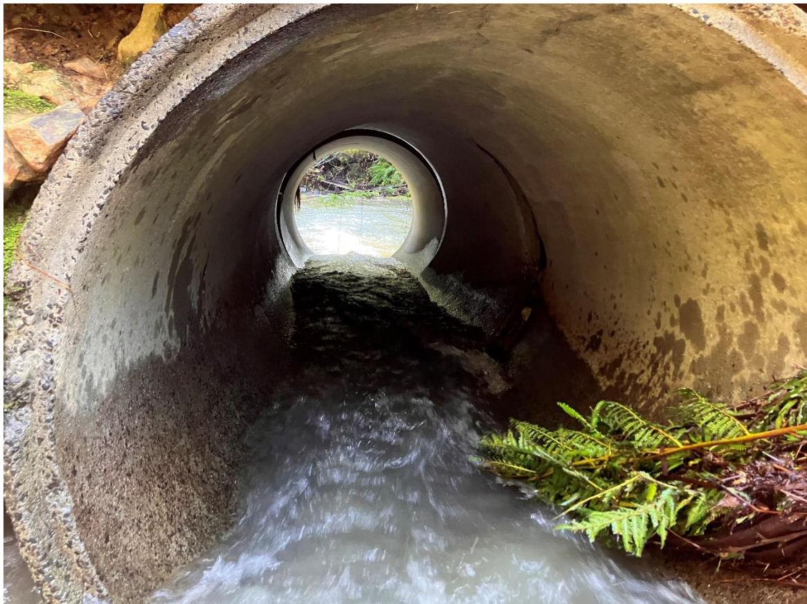
Dislodged pipes in existing culvert at C34032 taken: July 2025
