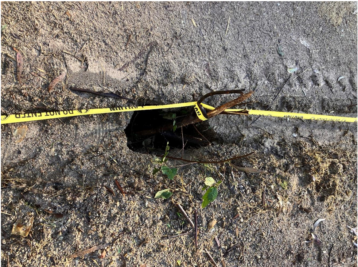
Example of void in road taken: July 2025
