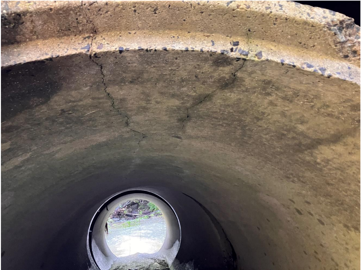
Existing cracks in culvert pipe taken: July 2025
