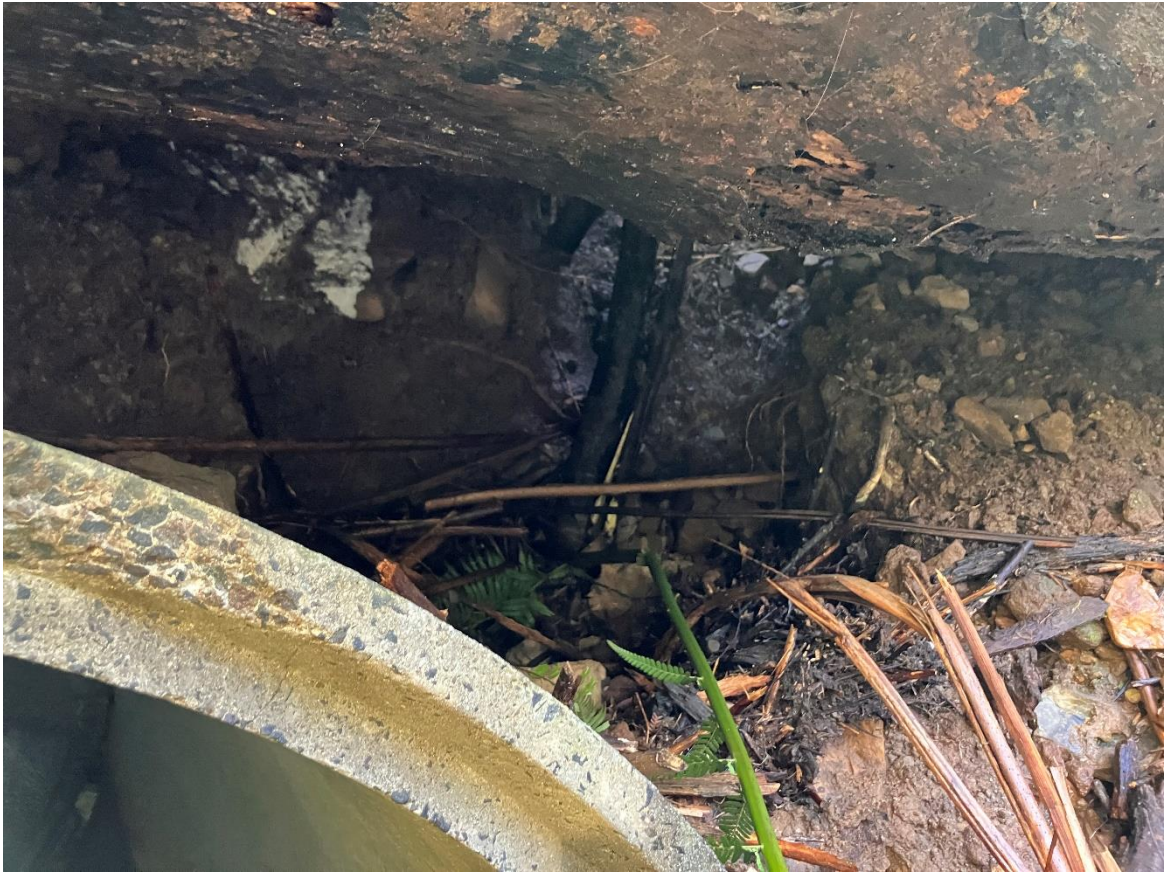
Example of void in road taken: July 2025
