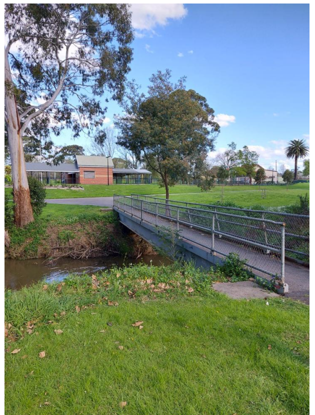
Image 7. At the north abutment looking southwest.
