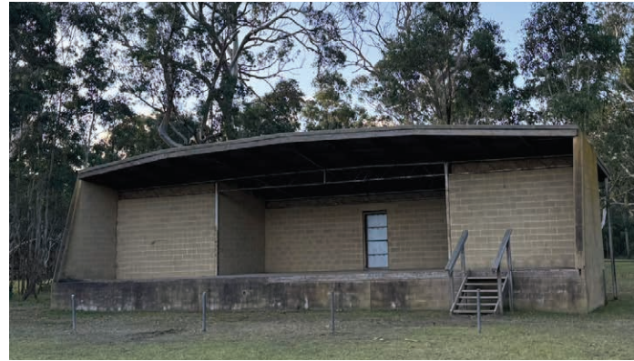
Event stage with fall from height risk. Does not provide adequate event acoustics. Power board unable to provide for event requirements
