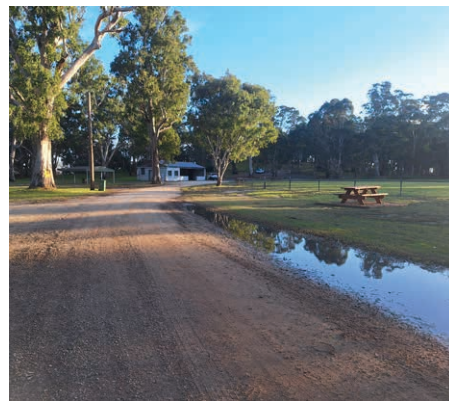
Poor drainage to western side of vehicle track to main picnic shelter
