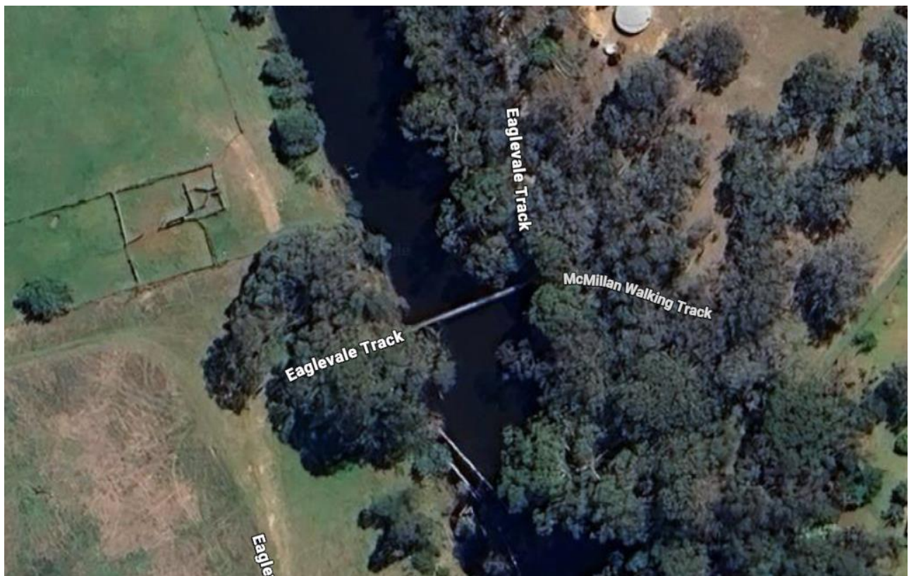
Figure 2: Aerial photo of bridge before January 2026 bushfire - Google
