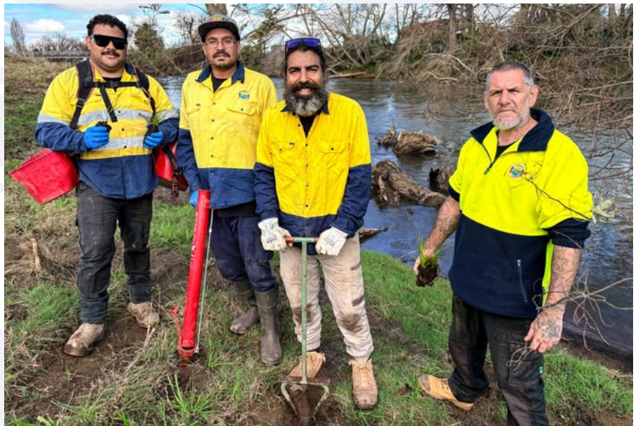
Natural Resource Management crew members Trey Parsons, Corey Jack, Phil Solomon and Ian Sullivan doing shore bank stabilisation works.
